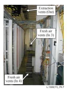
Figure II.7 – Rack aisle and air distribution system
