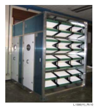
Figure II.10 – Filtration and humidification section
